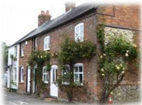
Terrace of cottages with no front garden
